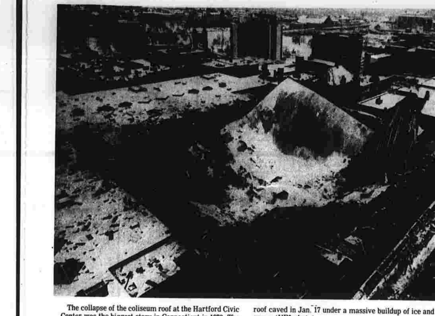
The collapse of the coliseum roof at the Hartford Civic Center was the biggest story in Connecticut in 1978. The roof caved in Jan. 17 under a massive buildup of ice and snow. (UPI photo)
